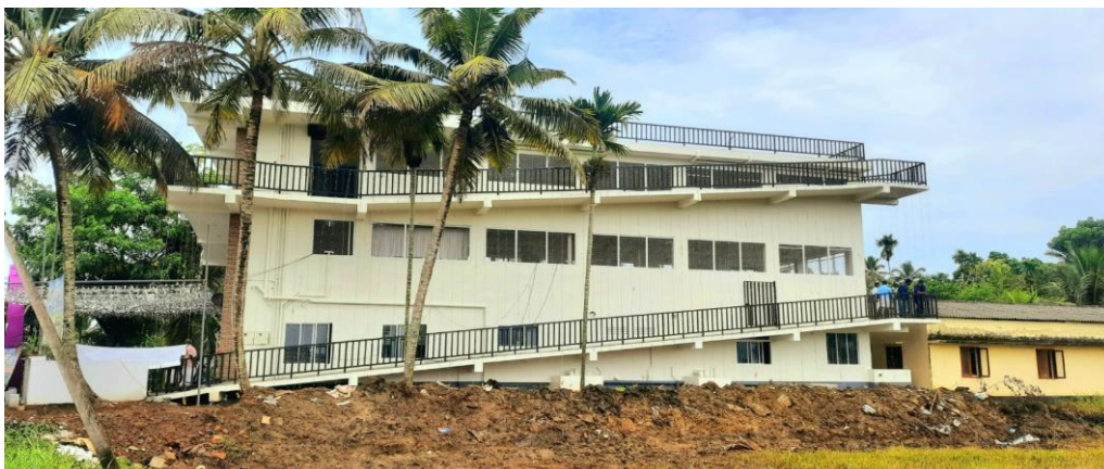
Elevated And Community Cattle Shed at Chempumpuram Dairy Co-Operative Society (Ltd No. 156(D) APCOS) - Inaugurated On 12.05.2022
